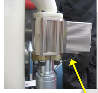
Sensor on pump discharge
