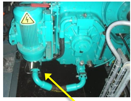
Sensor on pump intake
