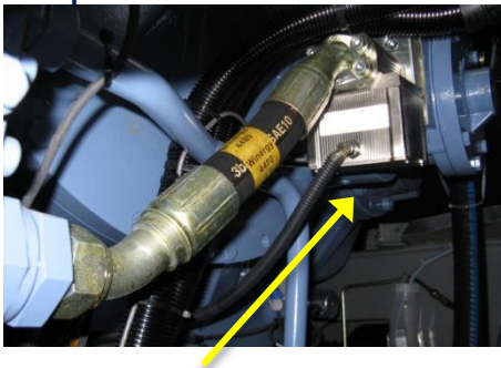
Sensor on pump discharge
